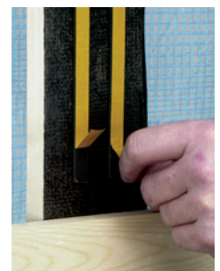
Pre-treatment of the backside / bonding side with Easy Clean Wipes
